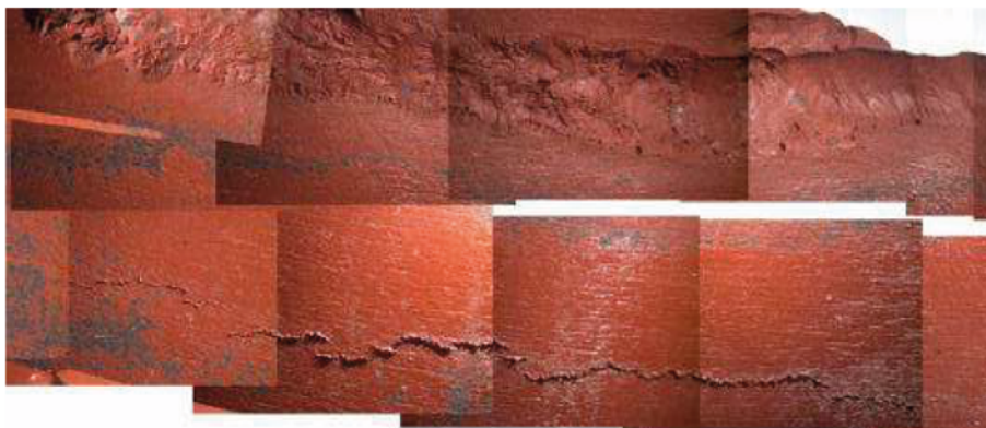
Figure 1: Replica mold with defect.
